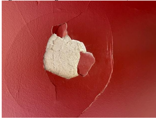
Figure 1: Second floor landing - exterior west wall
